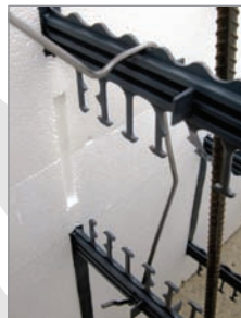
Vertical Clips in Place
