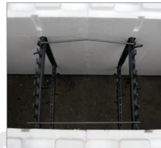
Horizontal Clips in Place
