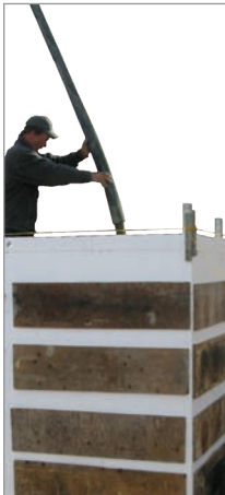
Some competitive ICF strap corners with lumber for strength during concrete placement.
